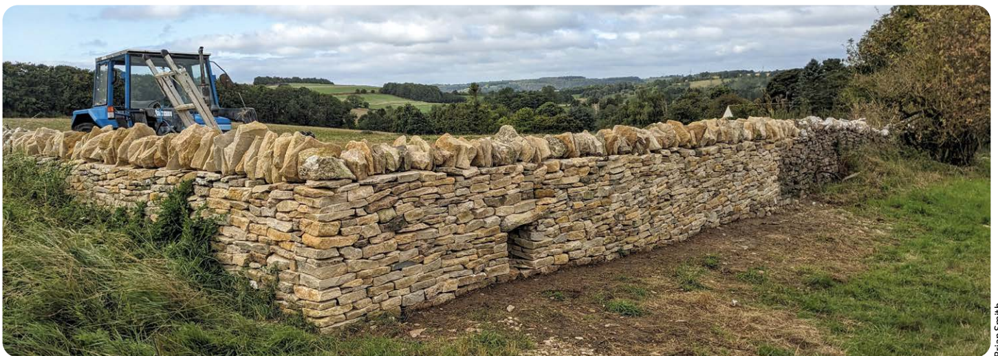
Rebuilt Cotswold stone wall at Compton Abdale.
