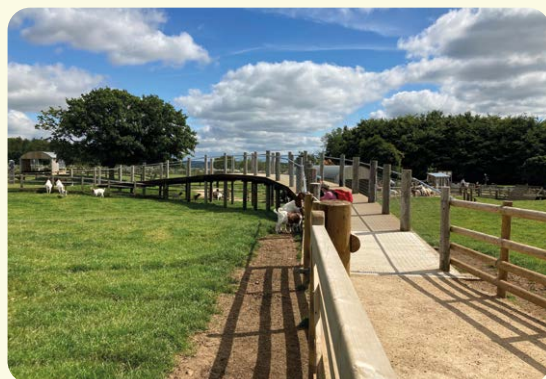
One of the raised walkways installed in the farm park.
