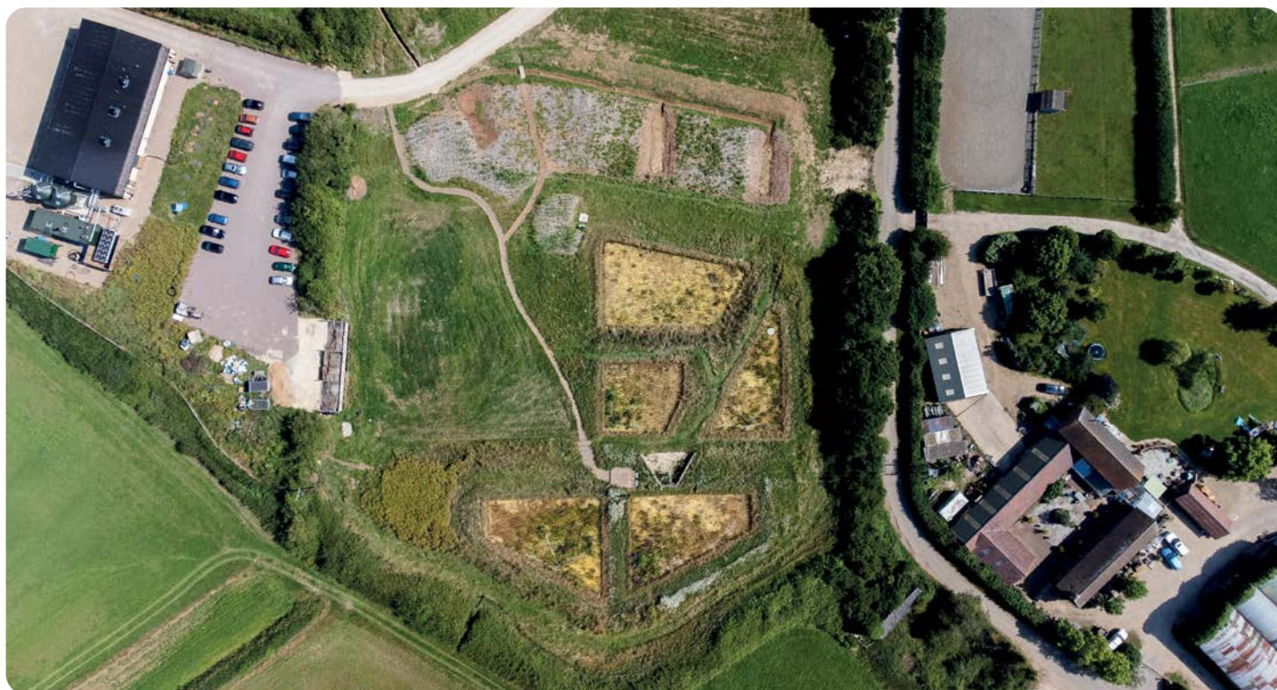
The wetlands treatment system from the air – showing the series of cells which break down the effluent.
