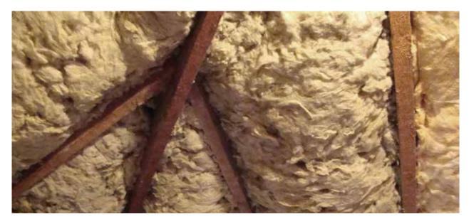
Wool based roof insulation.
