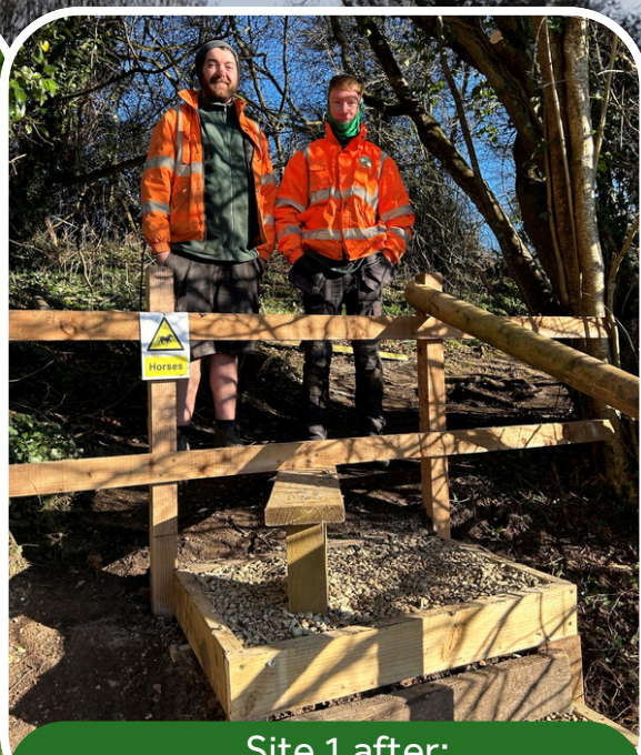
Site 1 after: New fencing, steps, stile and handrail
