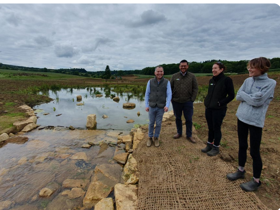
The Chipping Campden wetland project during construction in 2024
