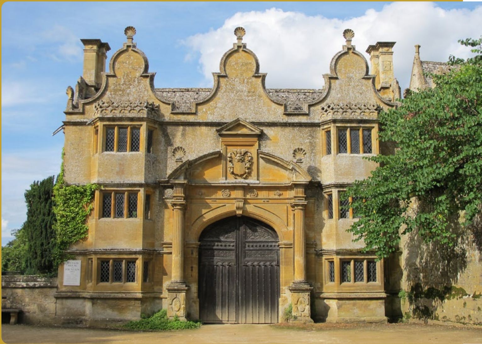
Golden hued stone is part of the charm of the gatehouse at Stanway House
