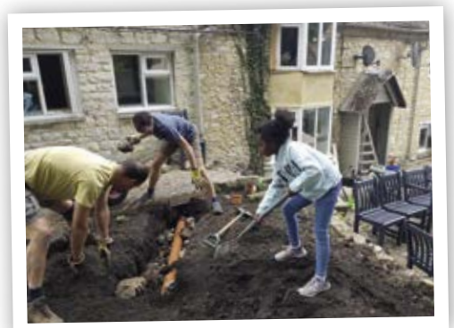
Volunteers got stuck into a range of jobs during the renovations
