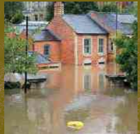
Previous flooding on Slad Road.
