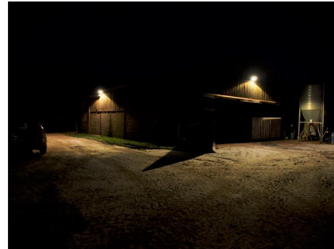
Figure 16 - An example of good farm lighting. Courtesy Mike Hawtin. North York Moors National Park. Note the correct colour temperature, direction, shielding and appropriate levels of illuminance for safe working.
